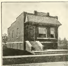
HAMILTON COUNTY TELEPHONE CO., AURORA
